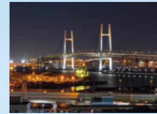
1989 Yokohama Bay Bridge
