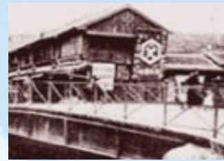
1868 Construction of Kurogane Bridge, Japan's first steel bridge
