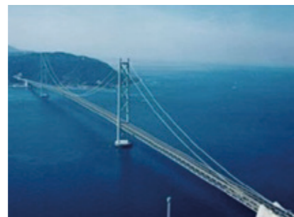
Akashi-Kaikyo Bridge (3,991 m) Japan Society of Civil Engineers "Tanaka Award"
