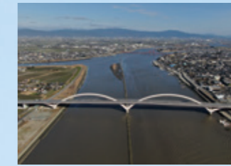
2021 Ariake Chikugo River Bridge
