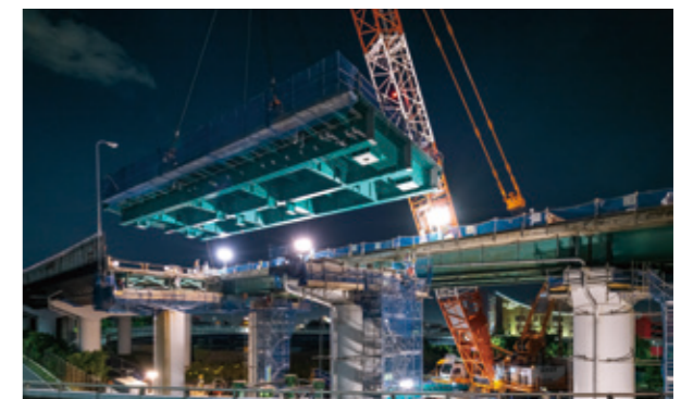
Suita Junction-Chugoku Expressway Ikeda Interchange Bridge renovation project (NEXCO West)
