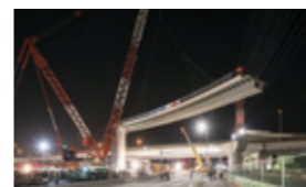
Tobishima Junction C Ramp Bridge
