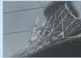
1958 Tokyo Tower under construction
