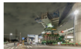
Tobishima Kiba Viaduct
