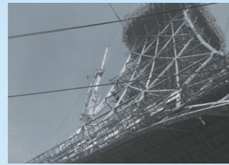
1958 Tokyo Tower under construction
