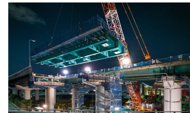
Suita Junction-Chugoku Expressway Ikeda Interchange Bridge renovation project (NEXCO West)
