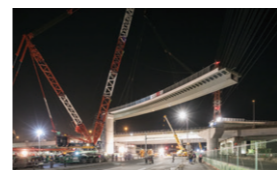
Tobishima Junction C Ramp Bridge
