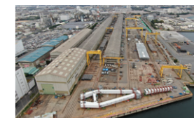
Chiba Works of MIYAJI ENGINEERING CO., LTD.
