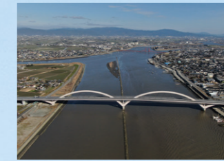
2021 Ariake Chikugo River Bridge
