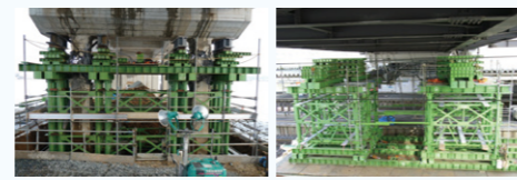
RC viaduct support pillar emergency response measures Natori connecting passageway
