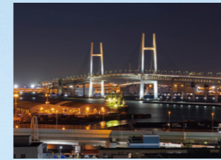
1989 Yokohama Bay Bridge
