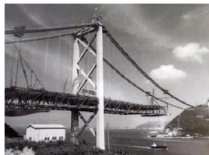
Kanmon Bridge (1,068 m) Japan Society of Civil Engineers "Tanaka Award"
