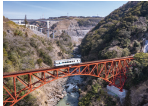
First Shirakawa Bridge
