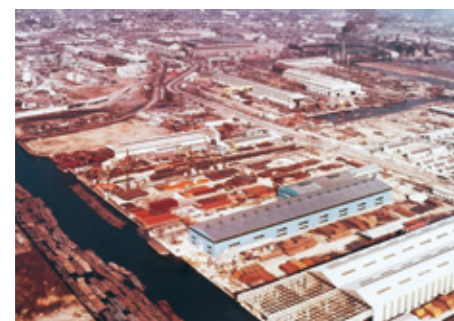
Suna-machi No. 3 Works
