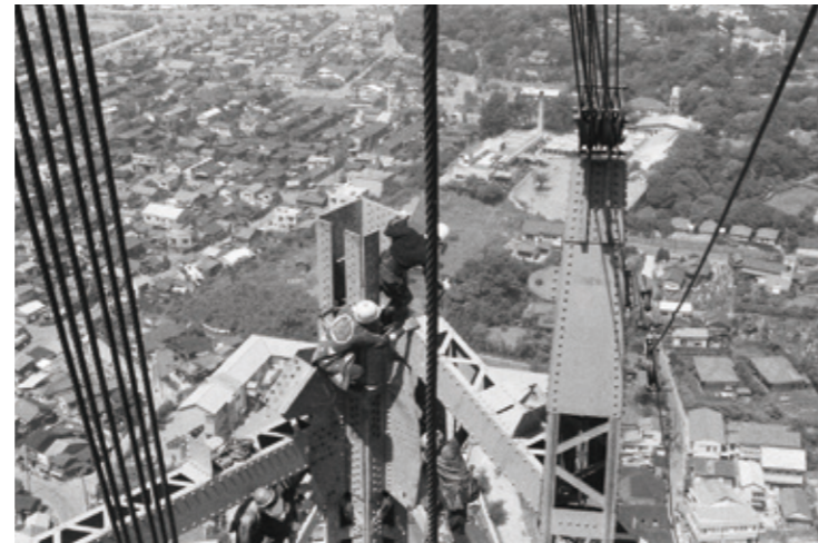
The construction of Tokyo Tower
