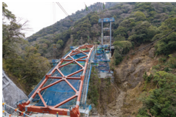
Cable crane erection
