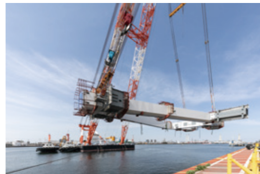
Preparing the main tower for shipping using a large FC
