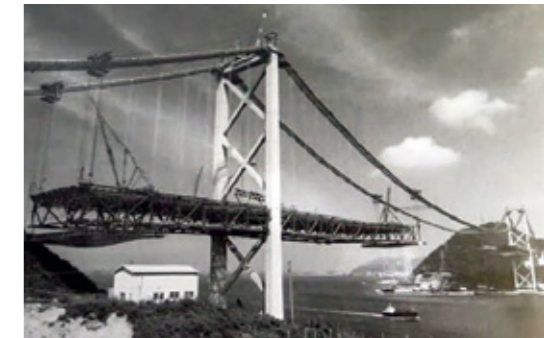
The Kanmon Bridge during erection
