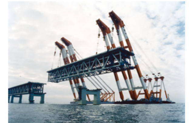
Large block erection using a large FC
