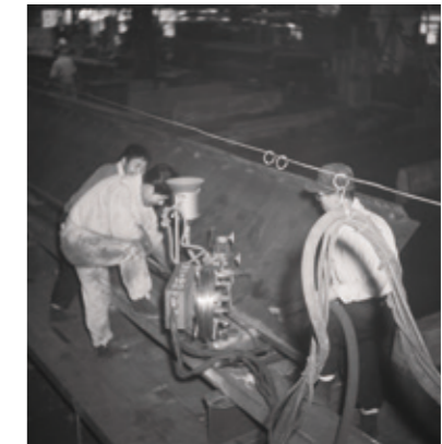
Work being done in the Hata Works
