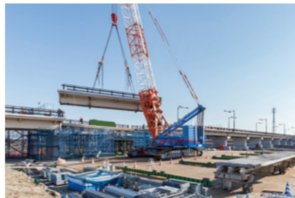
Removal using a crawler crane
