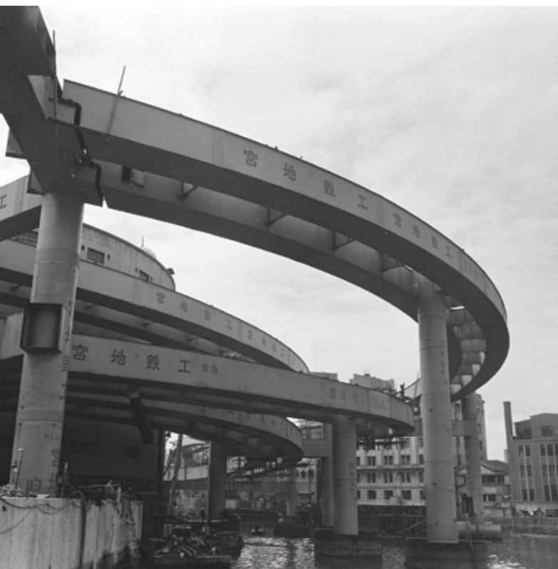
Edobashi Junction construction in progress
