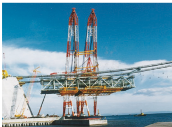
Large block erection of the Akashi-Kaikyo Bridge's stiffening girders
