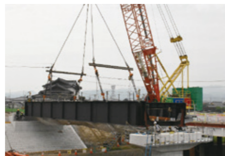
Large block erection using a crawler crane
