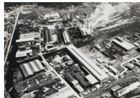
Suna-machi No. 1 and No. 2 Works
