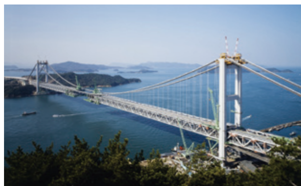
Shimotsui-Seto Bridge construction in progress
