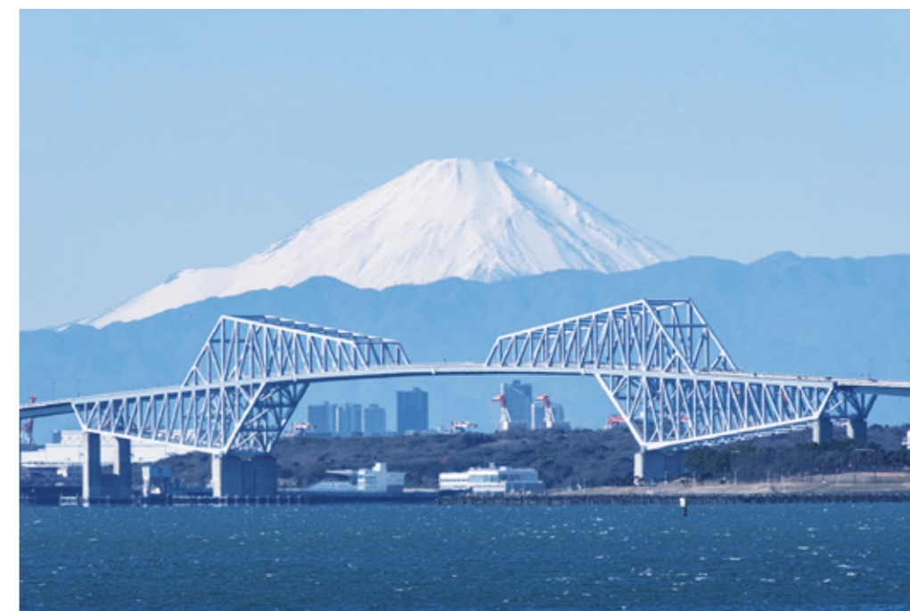
Tokyo Gate Bridge
