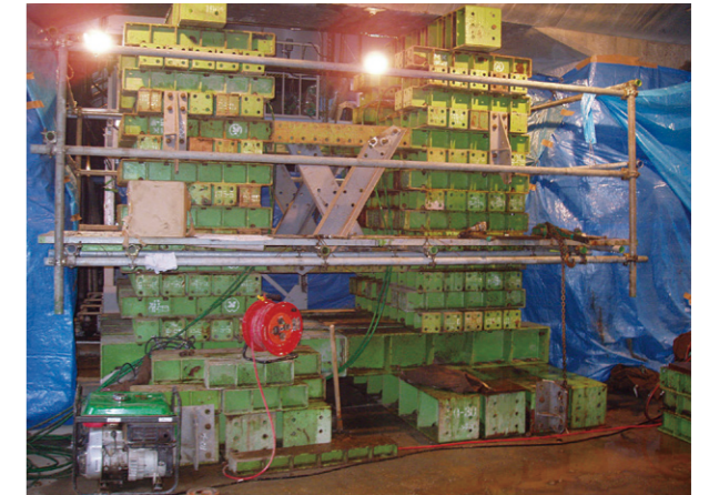
Joetsu Shinkansen’s RC viaduct support pillar emergency restoration measures
