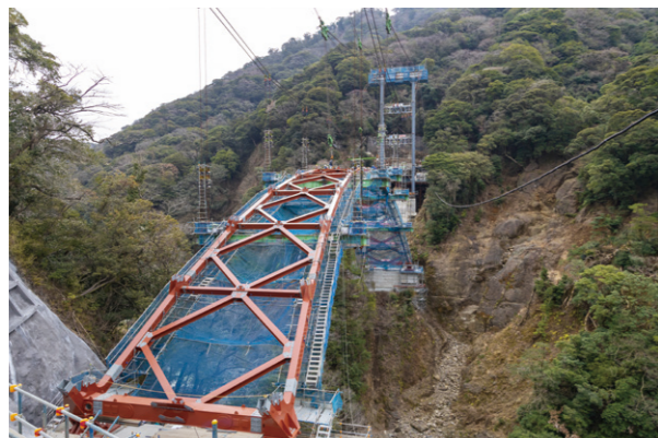
Cable crane erection
