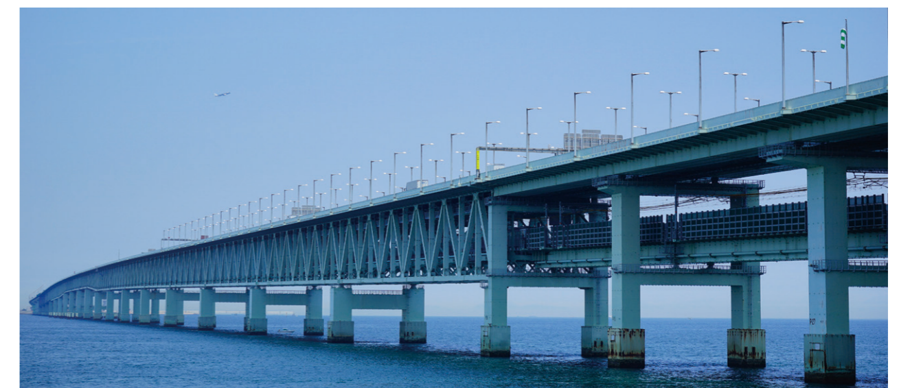
Kansai International Airport Access Bridge (Sky Gate Bridge R)
