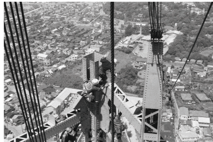
The construction of Tokyo Tower
