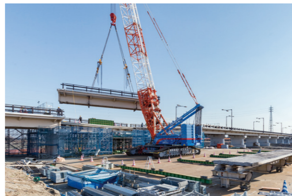
Removal using a crawler crane
