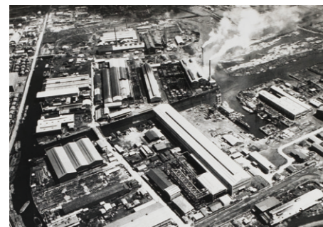
Suna-machi No. 1 and No. 2 Works
