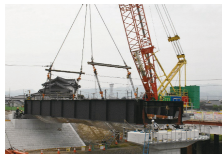
Large block erection using a crawler crane
