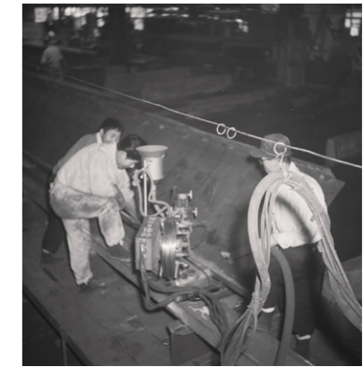
Work being done in the Hata Works
