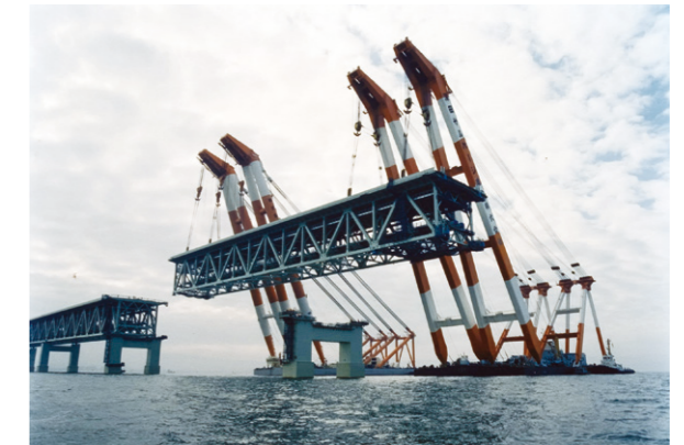
Large block erection using a large FC
