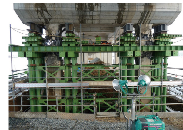
Tohoku Shinkansen’s RC viaduct support pillar emergency restoration measures
