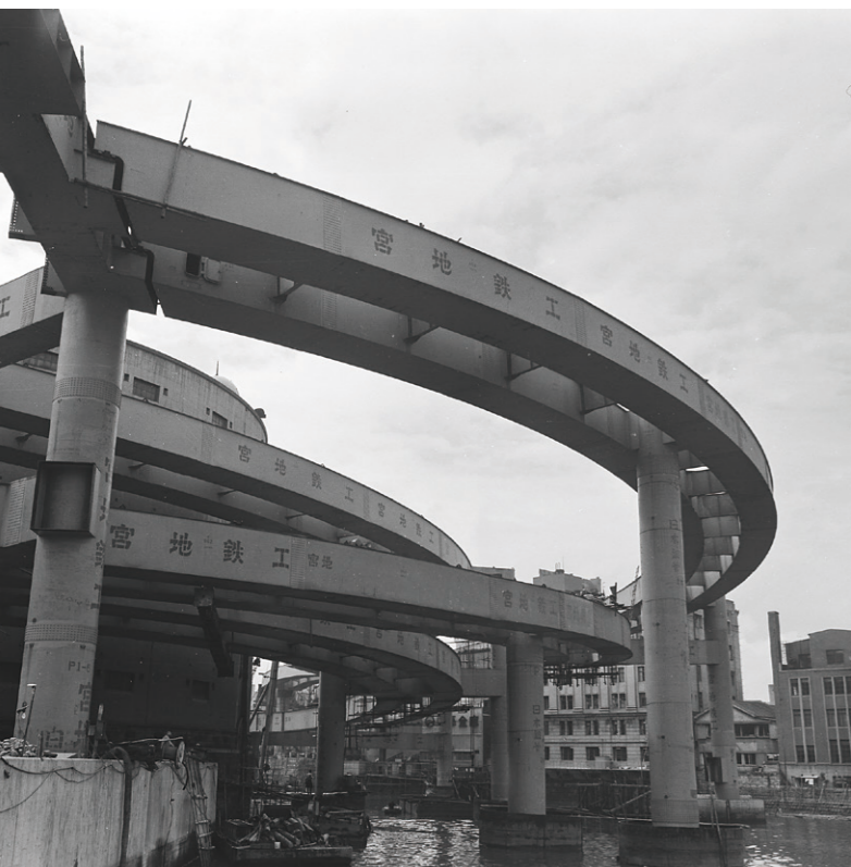
Edobashi Junction construction in progress
