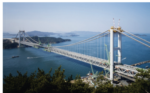
Shimotsui-Seto Bridge construction in progress
