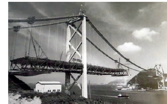
The Kanmon Bridge during erection
